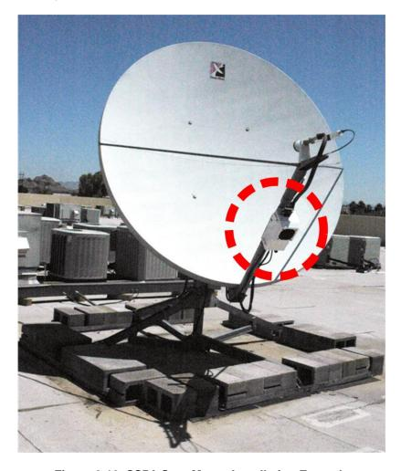
Figure 2-12. SSPA Spar Mount Installation Example
